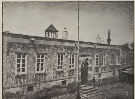
ERZROOM POST OFFICE, ACROSS THE STREET FROM THE BOYS' SCHOOL
